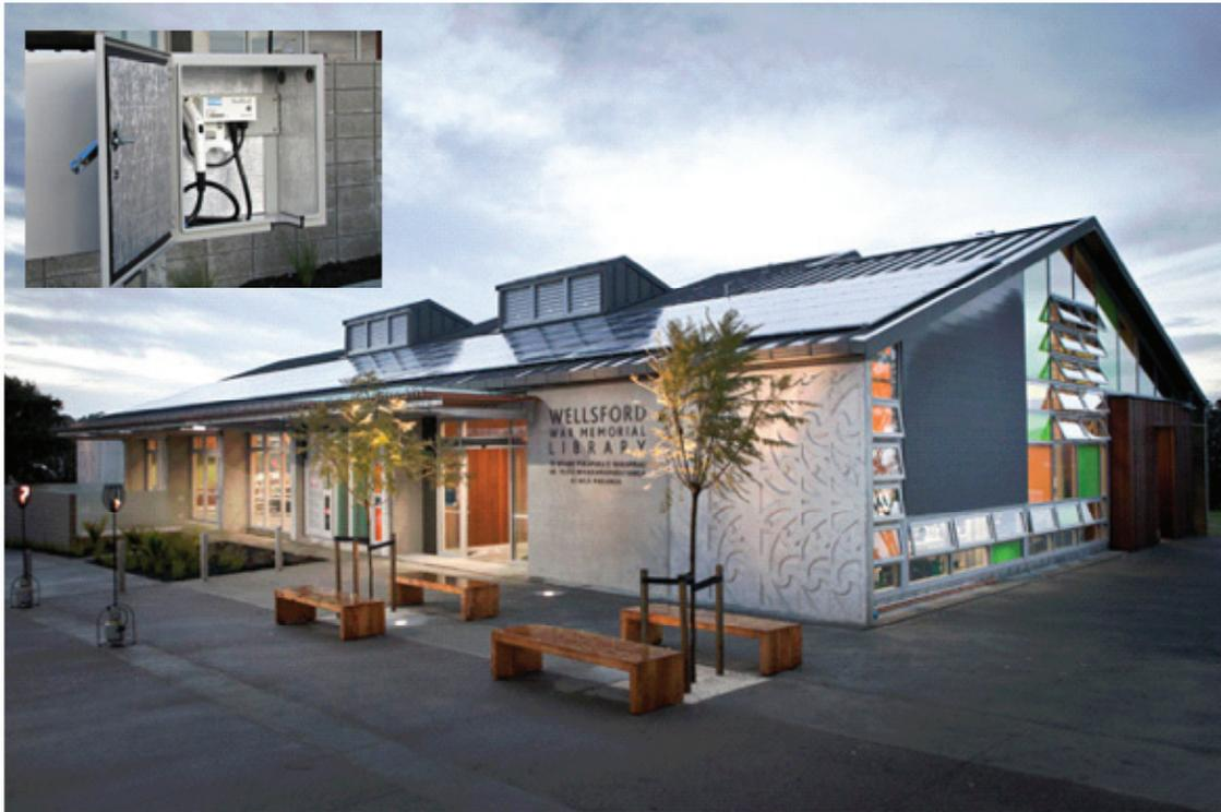
**Auckland Council's Wellsford library showing 29Kw solar PV array and insert of charging station.**
